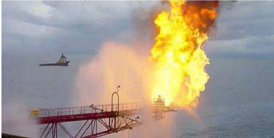
Woodside Petroleum's Chinguetti oil and gas platform off the coast of Mauritania.
