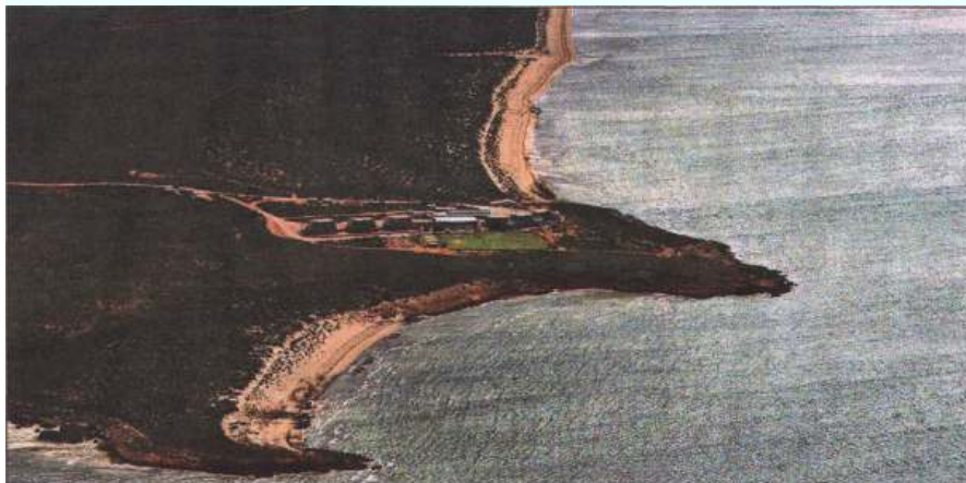
The latest plan for the Gorgon field is for a 15 million tonne a year project on Barrow Island.
