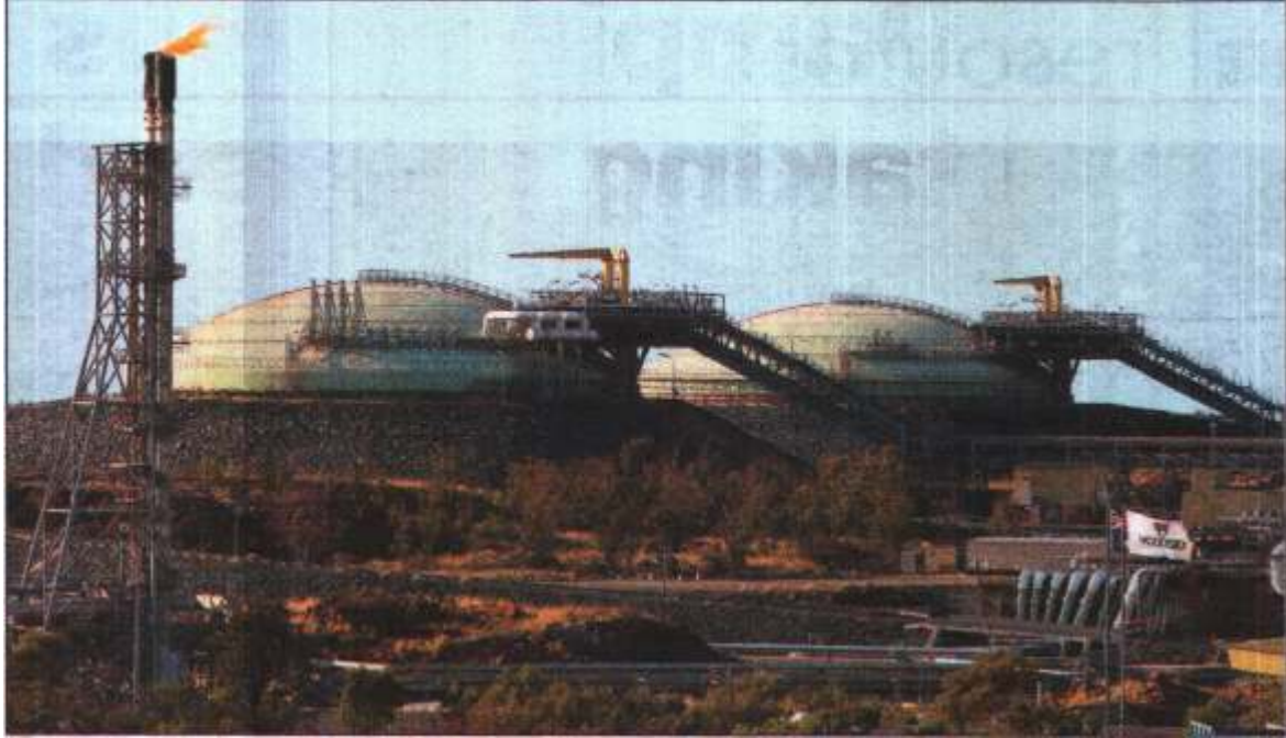
Woodside's LNG storage facilities on the Burrup Peninsula.
