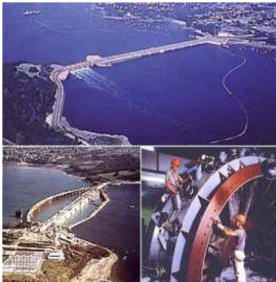
La Rance Tidal Power Station during and after construction (Image courtesy of Popular Mechanics ).
