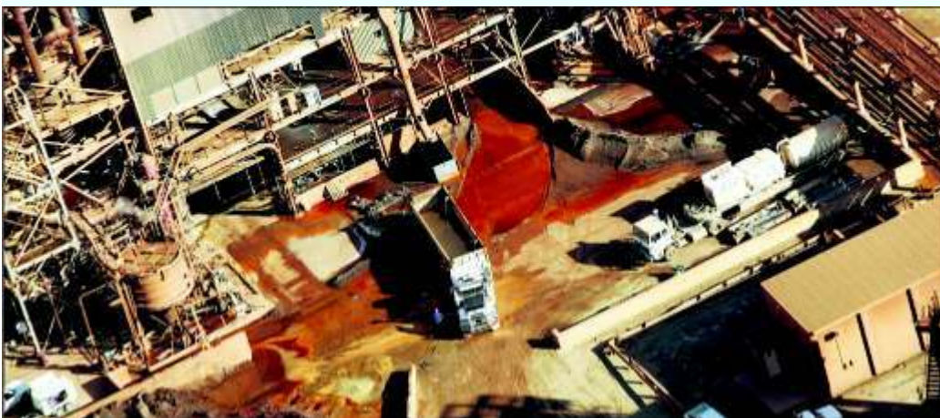
Power play: Turning bauxite into alumina requires huge amounts of power.
