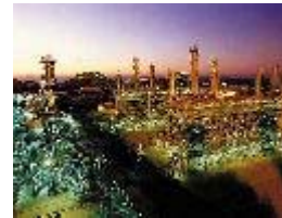
A previously completed train in the North West Shelf LNG project
