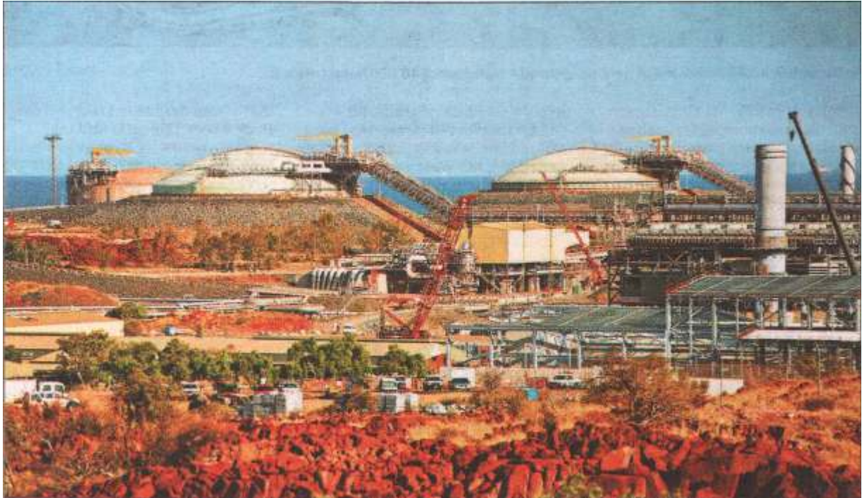
A Woodside gas processing plant on the Burrup Peninsula.
