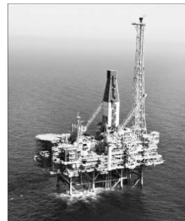
Submarine cables connect the platform to the shore-based processing plant.
